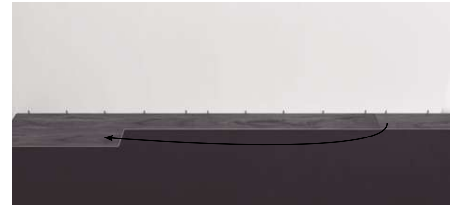
Step 6: Starting the second row the first plank should be a min length of 10" (254mm). Put a 3/8 (9,525mm) spacer against the wall and measure the last piece. If it is shorter than 10" (254mm) a new starter piece should be used. Insert at an angle into the previous row and tap (on the long side) it in using a tapping block till flat.
