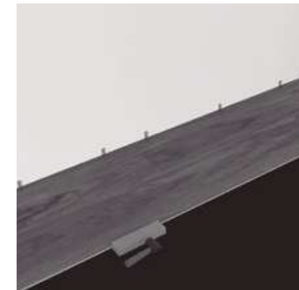
Step 9: After 2-3 rows. Adjust the distance to the front wall by placing spacers 3/8" (9,525mm) on the side walls and the end wall. Once the adjustment is done against the main wall, continue to install till the last row.
